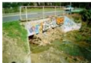
(d) Culvert Blocked by Tree Branches
