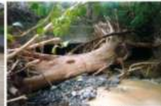
(c) Culvert Blocked by Tree Log
