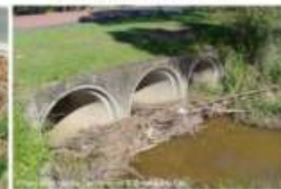
(f) Culvert Blocked by Tree Branches
