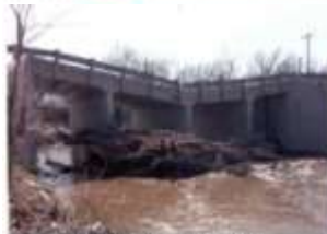
(a) Bridge Blocked by LW
