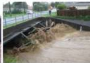
(b) Culvert Blocked by LW
